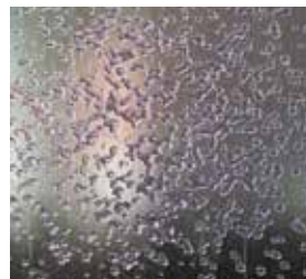
2. Gaps on surface increase risk.
